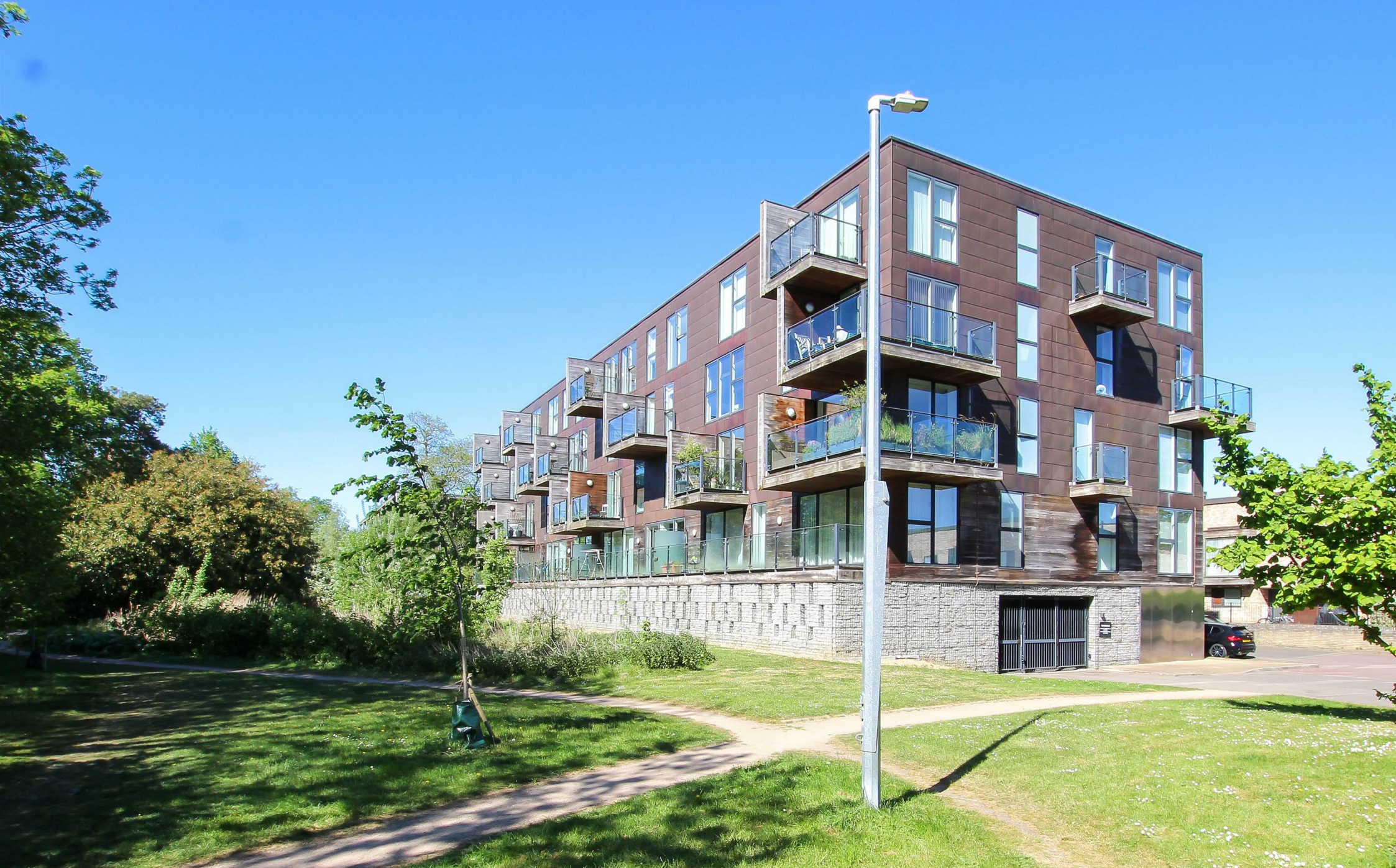
The Steel Building, Kingfisher Way, Cambridge, CB2 8BT
